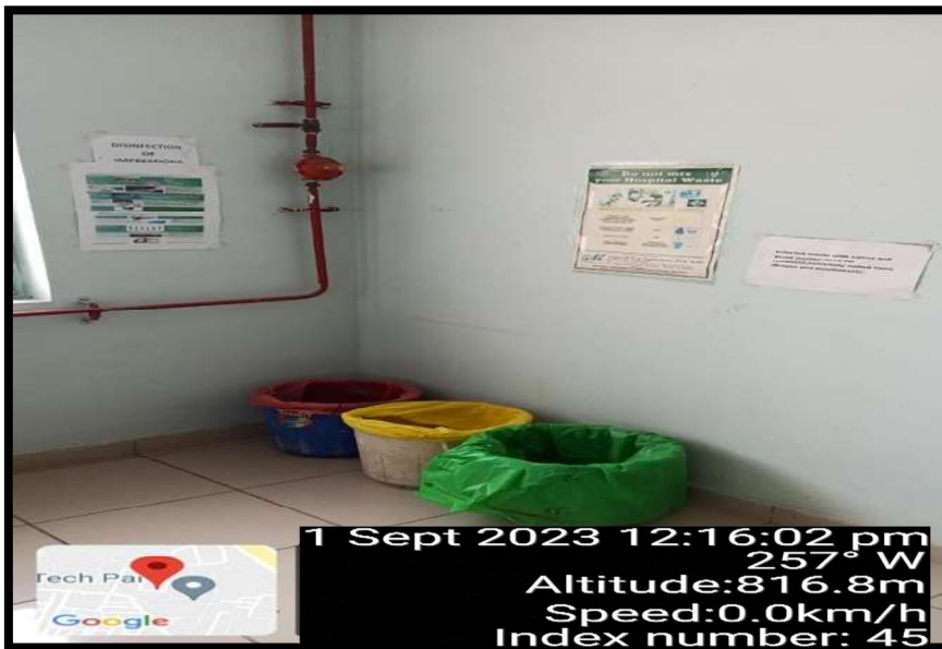
Dustbins for waste segregation (Dry/Wet/Plastic Waste) in the College
